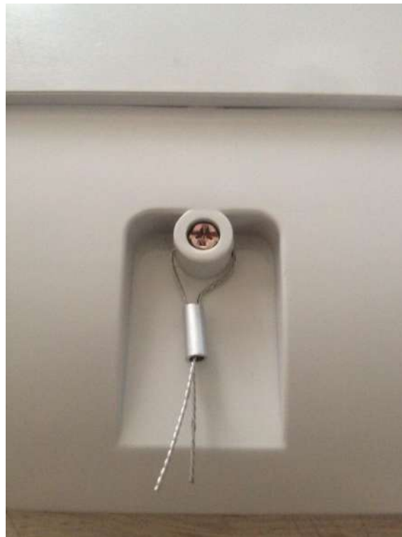
Figure .3.2.1 Terminal cover seal
